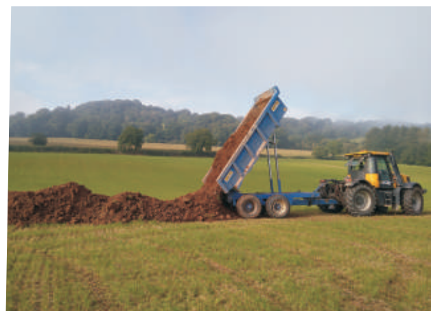
Soil from the creation of shallow ponds (scrapes) in a floodplain just 100m away is being used here to create a new bank. Photo Simeon Day.
